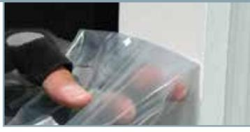
When installing other products such as HardiePlank® Lap Siding and HardiePanel® Vertical Siding with ColorPlus® Technology, leave the protective laminate sheet on the board during cutting and installation. Once the product is installed the laminate sheet should be removed.
