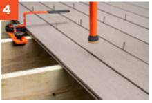
After fastening, lift up on the tool to return
